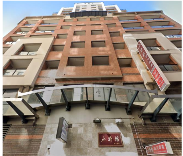
Picture 2 – APX Darling Harbour at 2-8 Dixon Street, Facing East
