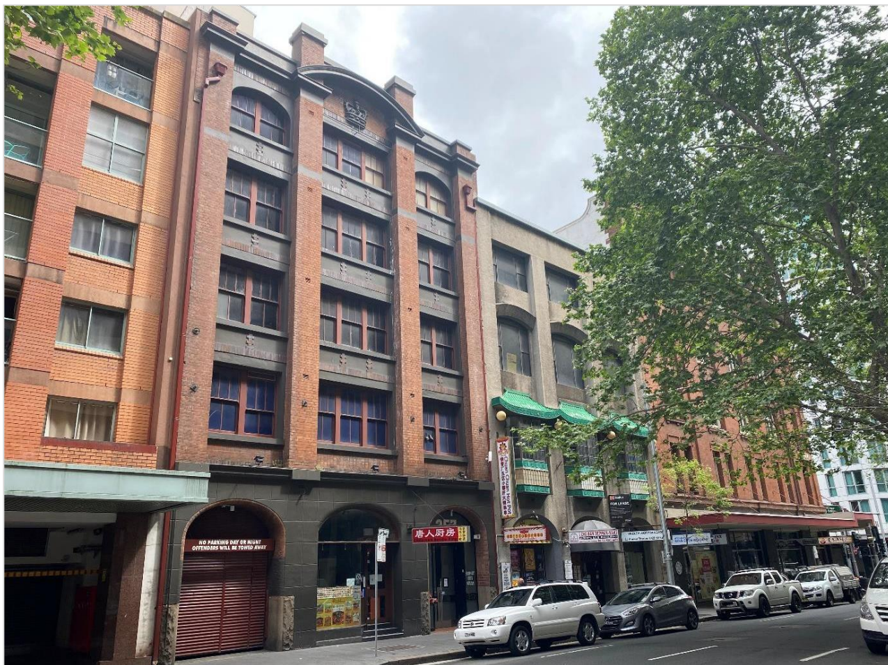
Figure 2 – Existing Image of Sussex Street Frontage, Facing North-West
